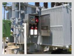
Continuously circulating online filtration of dielectric oil has proven to be a cost-effective means of combating load tap changer problems. The tap changers with permanent installation of our TCF system can enjoy obtain the following benefits:
